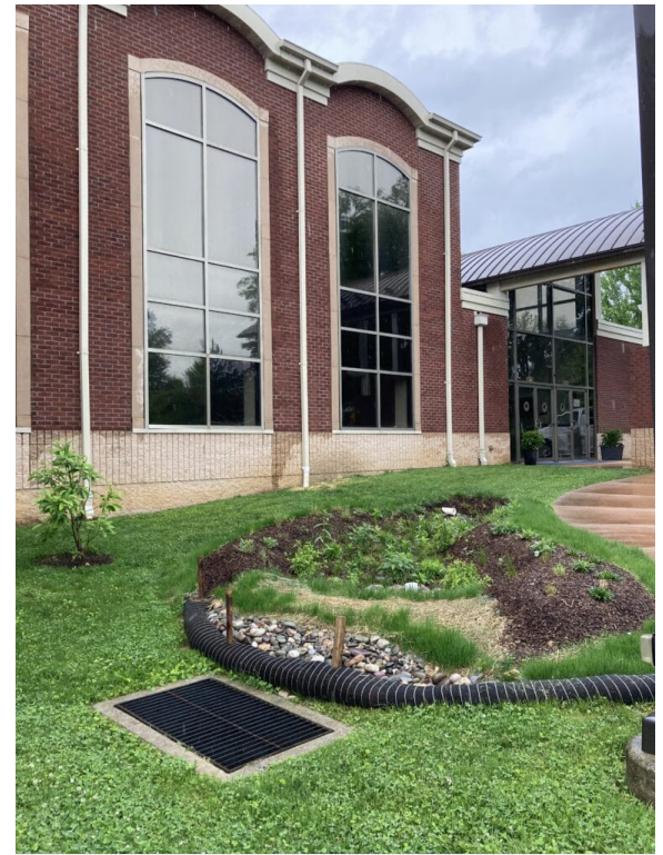
The rain garden at Bright Side Opportunities Center with soak up stormwater runoff and eliminate impervious surface. (Photo: Alliance for the Chesapeake Bay)
