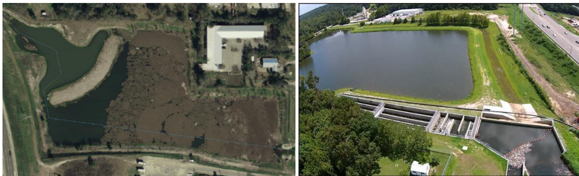
Figure 3. Original Weems Pond (left) and Upper Lake Lafayette Nutrient Reduction Facility (right)
