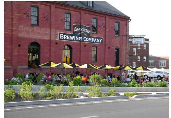
Patio rain garden and vegetated curb extension outside Lancaster Brewery. (Photo: City of Lancaster)
