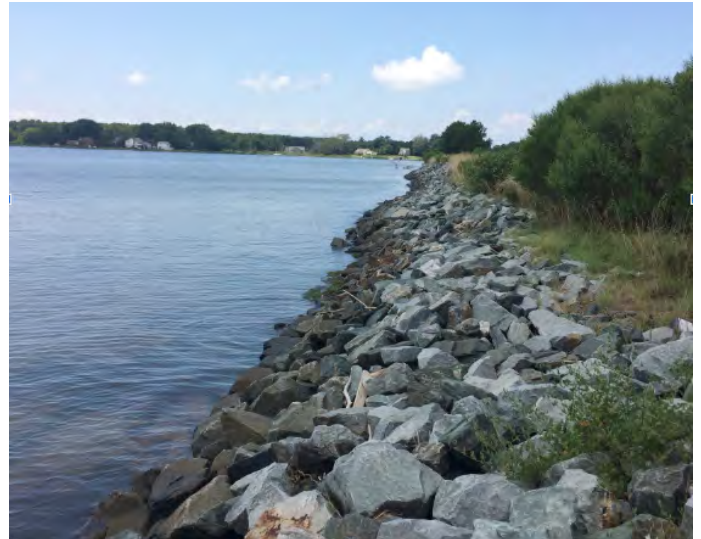
An on-shore stone revetment in Talbot county. (Rebecca Swerida)
