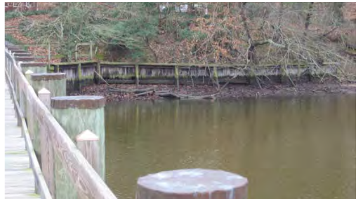
Timber bulkhead with base sediment accumulation visible at low tide in Talbot County. (Rebecca Swerida)
