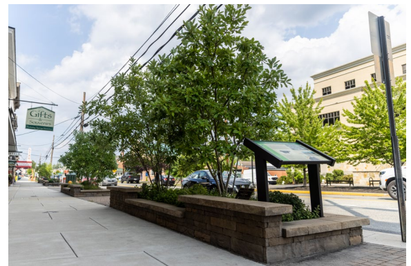
Tree boxes and permeable pavers divert stormwater from the town's business zone.
