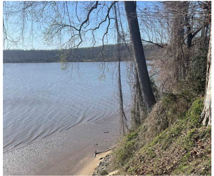
Large trees are at risk of falling and destabilizing the river bank.
