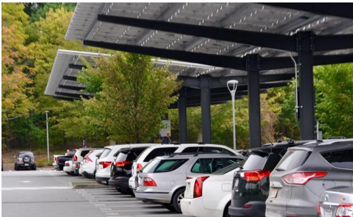
Parking lot integrates solar structures that provide multiple benefits including power, cooling and stormwater conveyance.
