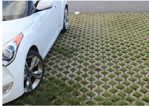
5. Parking surface such as gravel (existing) or pervious pavers to reduce runoff
