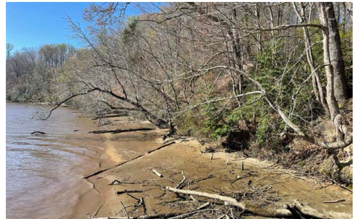
Erosion and wave action is destabilizing portions of the river bank.
