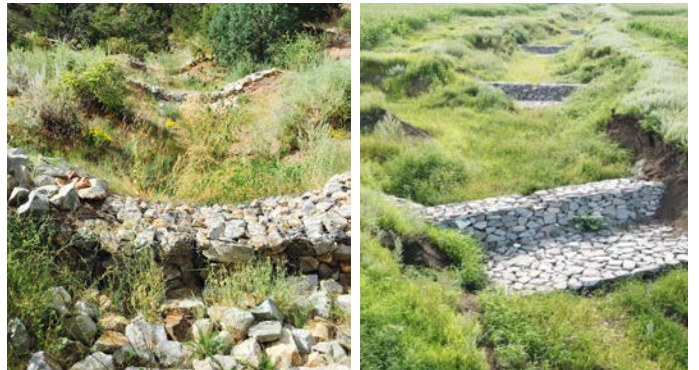
Check dams made of stone or gabion baskets slow water flow and stabilize soil while allowing water to soak into the soil and support vegetation..
