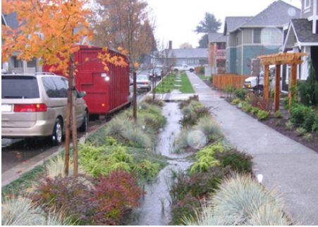
1. Planted swale along Leonards Lane to capture street runoff and buffer sidewalk
