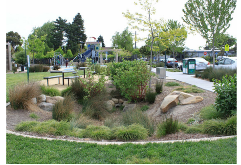
3. Planted swale to capture surface water and oil from parking area
