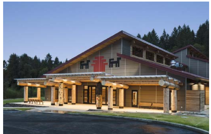
The design of the Skokomish Community Center provides a new gathering and recreation place for the Skokomish Tribe that expresses and celebrates the culture and traditions of the Tribe. The building was designed to be as "green" and sustainable as possible within the constraints of budget and the site conditions.
