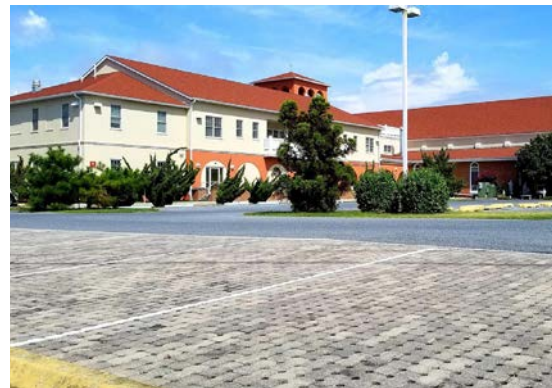
Permeable parking areas including trees and planted swales reduce stormwater runoff.
