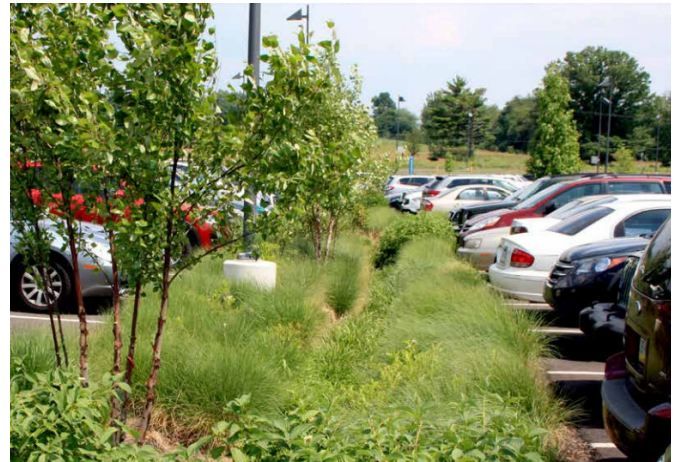
Planted swales in the parking lot capture and treat stormwater runoff.
