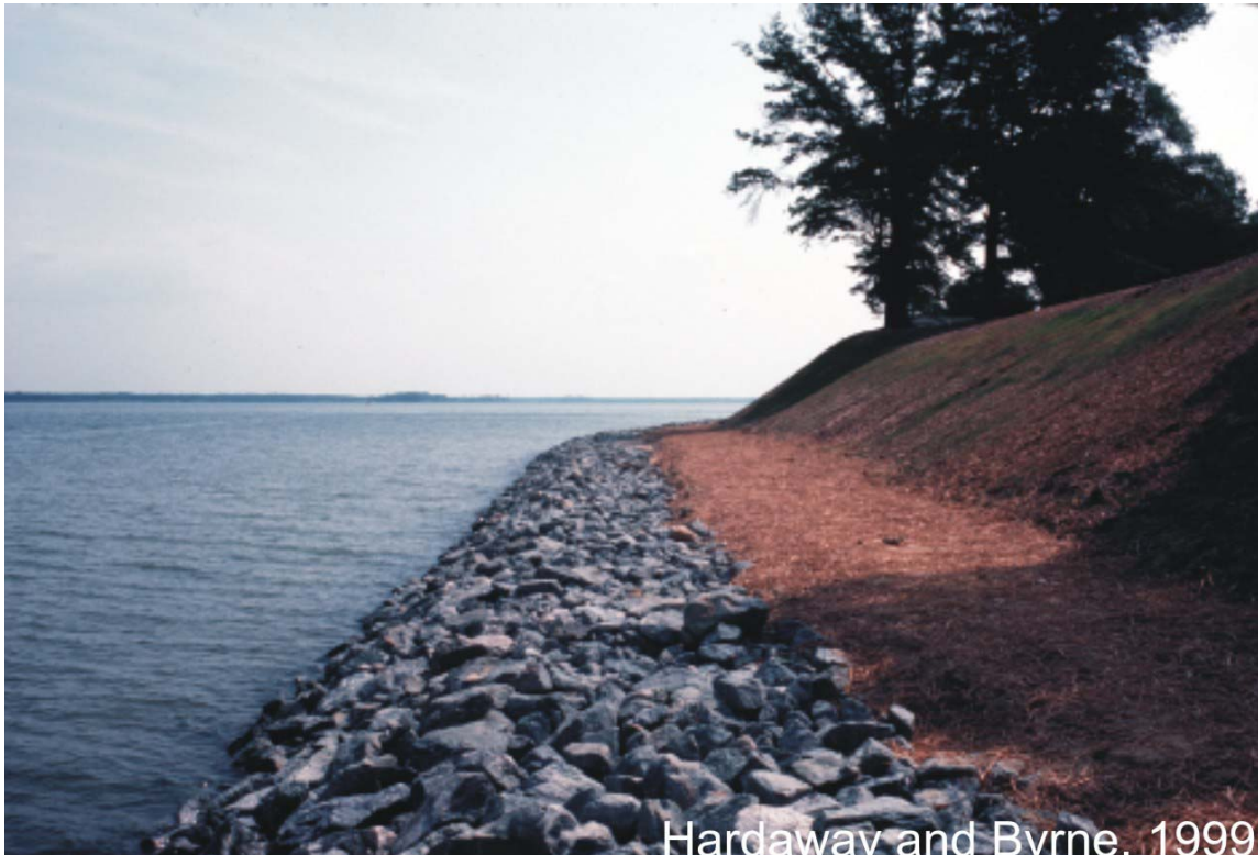
Figure 12 Stone revetment on the Potomac River, Virginia.
