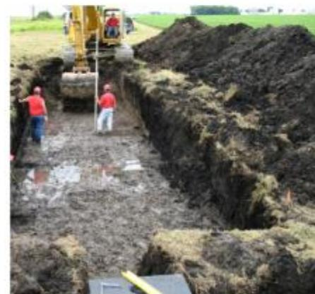
Excavating the pit for bioreactor installation.
