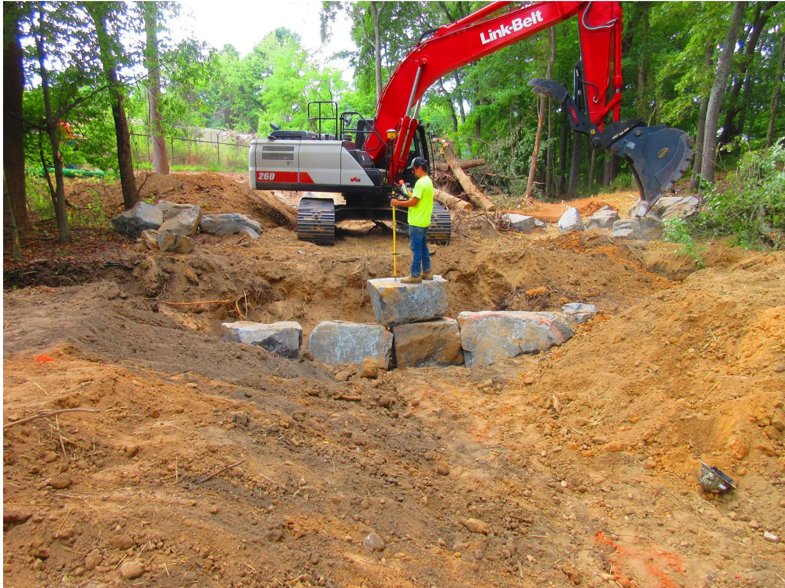
Installation of a Cobble Stone Weir
