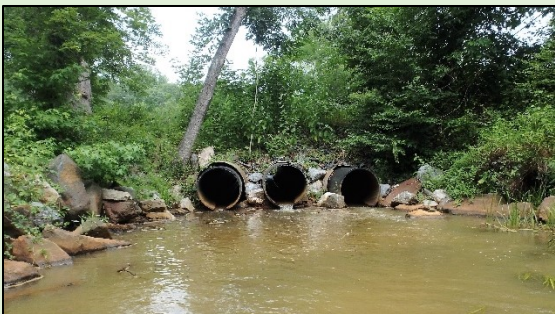
Original triple pipe culvert at Rutland Road
