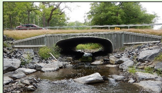
Replacement bottomless culvert at Douglas Road (Photo credit: Betsy Trometer, USFWS)
