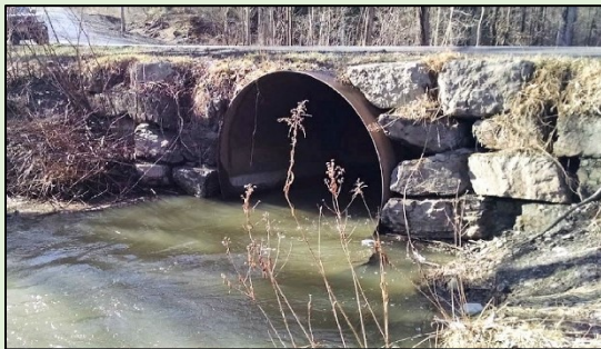
Original steel pipe culvert at Douglas Road (Photo credit: unknown, T.G. Miller, P.C.)
