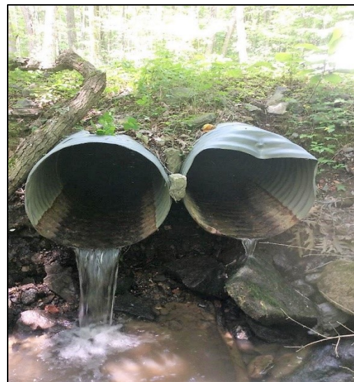
Undersized culverts can become a barrier to aquatic organism movement long before they become an issue for public safety and infrastructure. (Photo credit: Seth Moessinger, Trout Unlimited)
