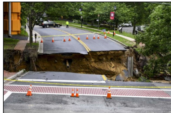
Collapsed roadway in Ellicott City, MD due to flooding (Photo credit: Katherine Frey, The Washington Post)
