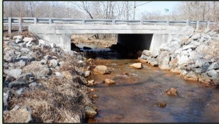
Replacement slab bridge at Rutland Road
