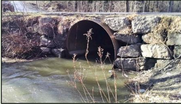
Original steel pipe culvert at Douglas Road
