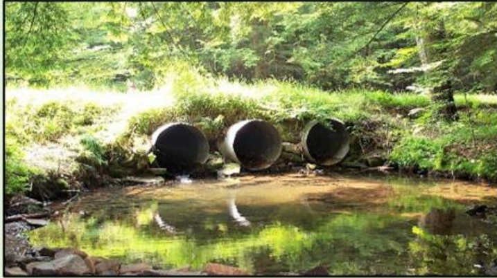
Original triple pipe culvert at USFS Road 116/2 (Photo credit: Brent Pence, USFS)
