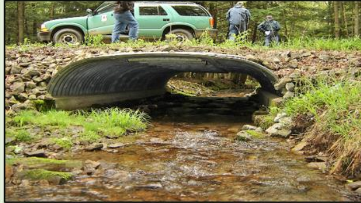
Replacement bottomless culvert at USFS Road 116/2 (Photo credit: unknown, USFS)
