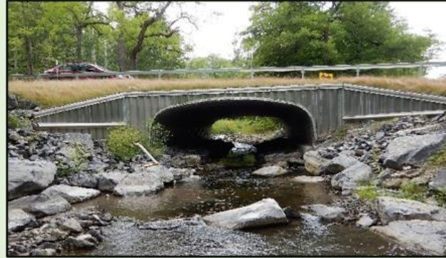
Replacement bottomless culvert at Douglas Road
