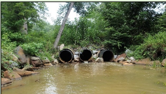
Original triple pipe culvert at Rutland Road
