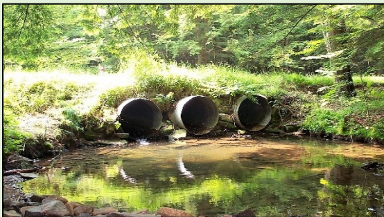
Original triple pipe culvert at USFS Road 116/2 (Photo credit: Brent Pence, USFS)
