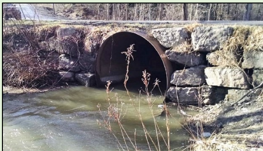
Original steel pipe culvert at Douglas Road
