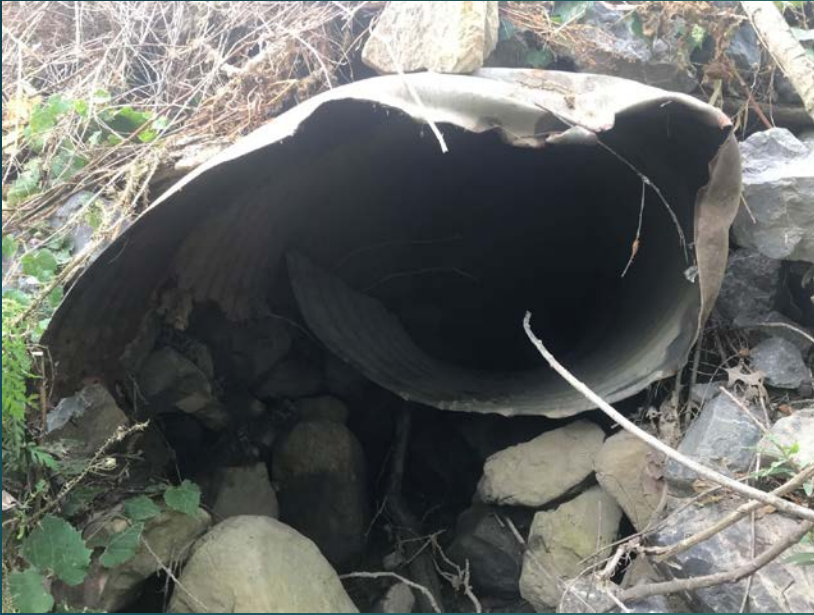
Mill Creek Headwaters: culvert inlet collapsed and was badly deformed
