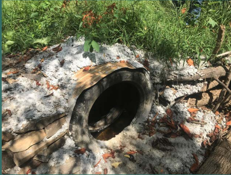
Mill Creek Headwaters: culvert constructed from tires, logs, plywood, and concrete
