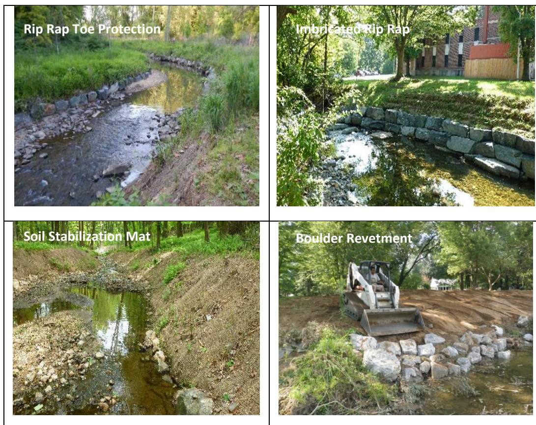
Figure 5. Examples of “creditable with limits” bank armoring practices
