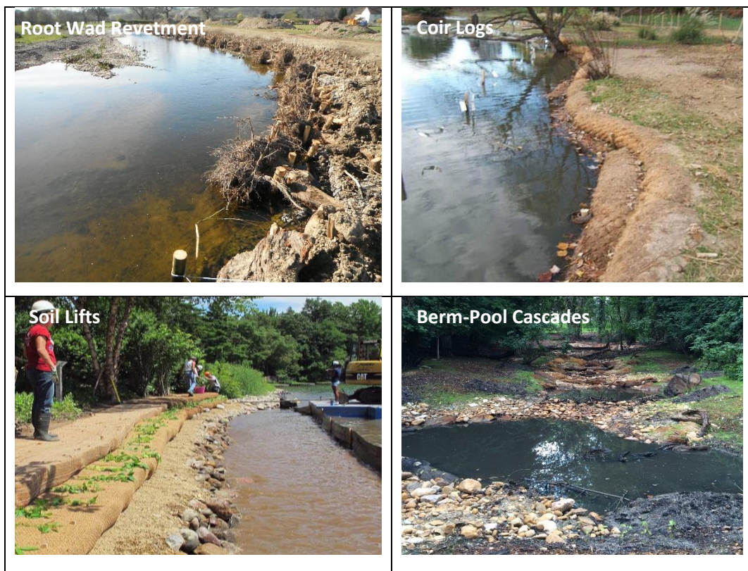
Figure 6. Examples of “creditable” armoring practices.
