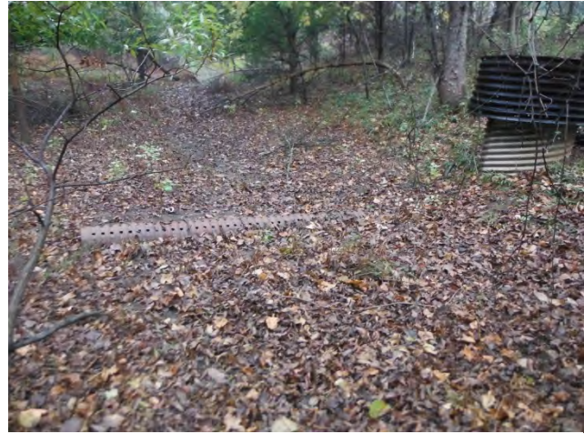
Figure 4 - Hunt Ridge pond bottom facing west at low flow perforated Outlet pipe.
