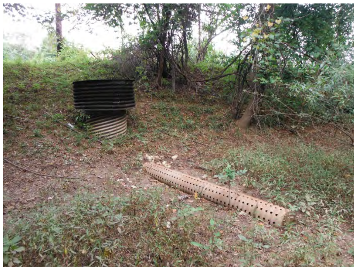
Hunt Ridge: Riser/low flow outlet pipe
