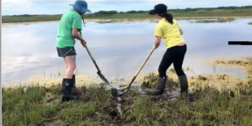
Runnel excavation by hand in summer of 2018
