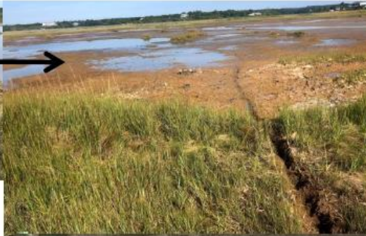
Runnel excavation by hand in summer of 2018
