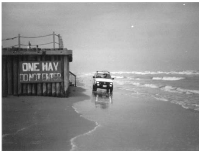
Photos 16 to 18. Shoreline armoring can make vehicular and pedestrian access along the shore impractical. Top left: a seawall protecting some high-rise buildings along the Gulf of Mexico on North Padre Island prevents automobile traffic on the beach (March 2010). Top right: At first, traffic was restricted to one-way (March 1998). Bottom: a stone revetment makes walking along the shore impractical north of Surfside, Texas (May 2003). Photo source: ©James G. Titus, used by permission.
