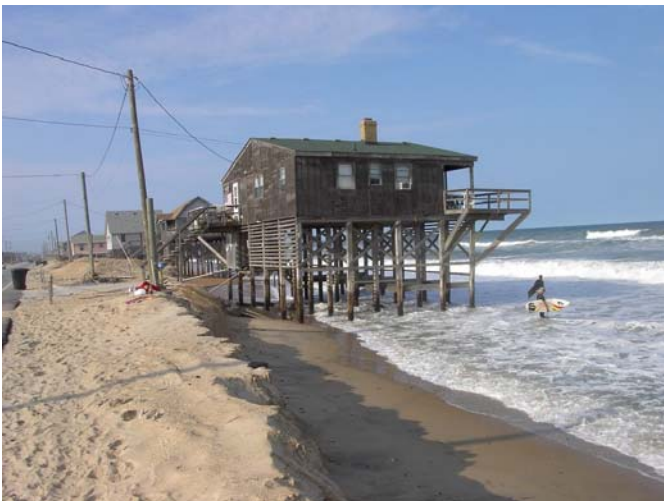
Photos 1 to 4. Few landowners choose to give up their homes to a rising sea. Top left and right: A home on pilings in front of shore protected by a stone revetment (left) and two homes protected by seawalls (right) on land extending into the Gulf of Mexico, along Bluewater Drive north of Surfside, Texas (May 2003). Bottom left: a home on pilings on an eroding beach at Kitty Hawk, North Carolina (October 2002) Bottom right: homes behind a bulkhead whose toe is protected by a stone revetment at North Beach, Maryland (September 2008). Photo source: ©James G Titus, used by permission.
