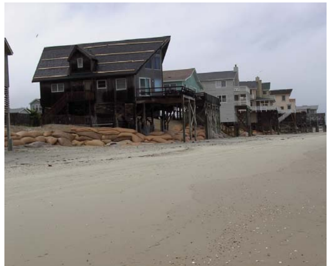
Photo 21. Geotextile sand bags along the beach in Nags Head, North Carolina. Although the homes were on pilings, the geotextile sandbags were needed to protect the septic tanks. (June 2003). [Photo source: ©James G. Titus, used by permission].
