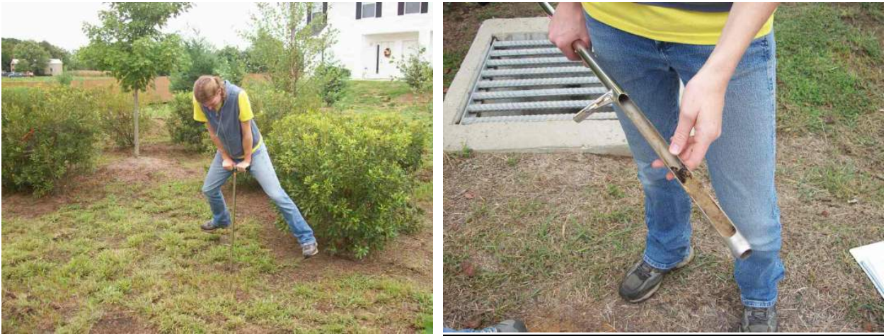
Figure 19. Compacted bioretention soil (left) with high clay content (right).
