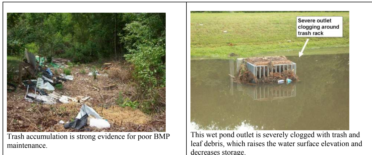
Figure 23. Common maintenance issues identified through the study.
