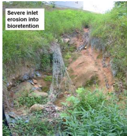
Figure 23 (continued). Common maintenance issues identified through the study.
