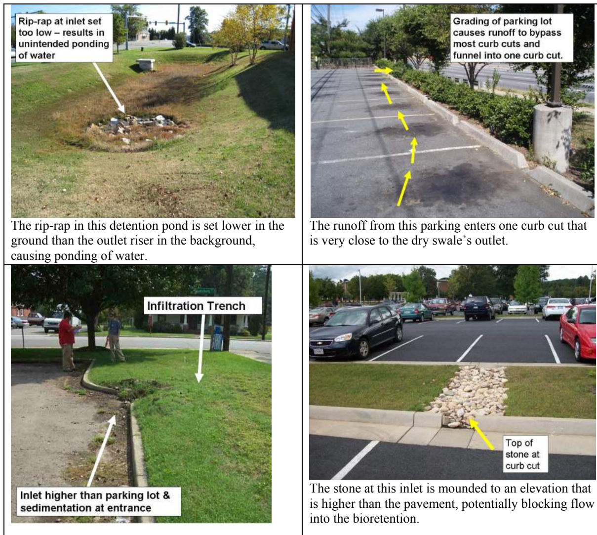
Figure 18. Examples of poor design features associated with grading and elevations.
