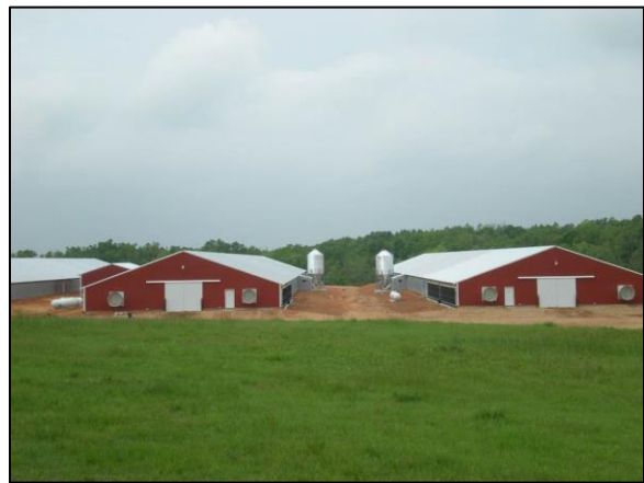
Figure 4. Broiler production houses.
