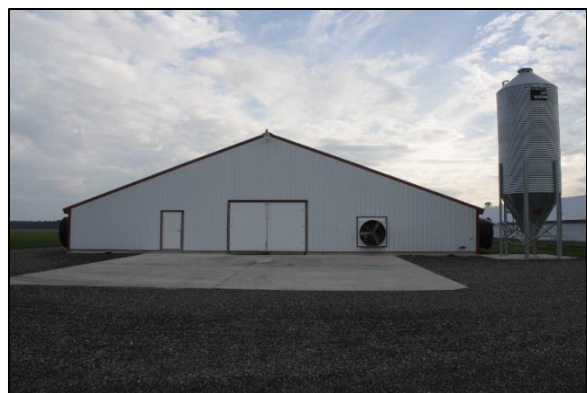
Figure 5. HUA protection outside a broiler house.
