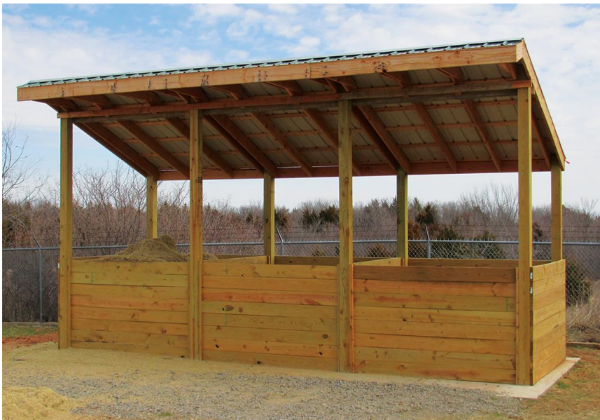
Figure II.3.4. “Three Bin” mortality composter (Langston University).
