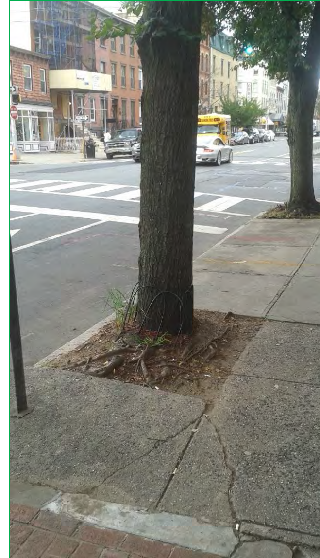
This tree is in too small a planting area and the sidewalk is starting to crack.
