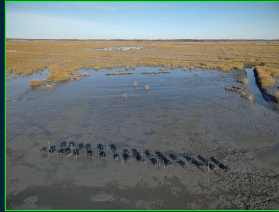
MarshGuard array raising elevation for SAV planting in NJ
