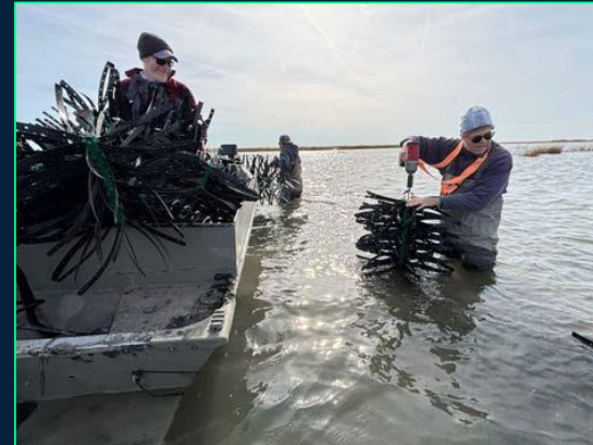
MarshGuard array raising elevation for SAV planting in NJ
