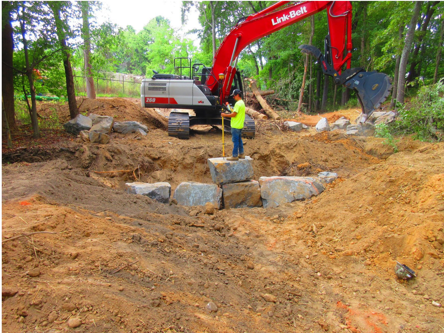
Installation of a Cobble Stone Weir
