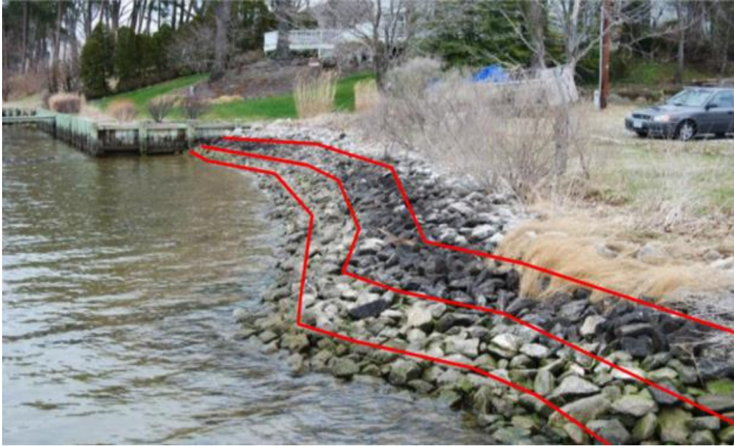
Figure 5. Image of rock discoloration indicating different tidal zones. The upper, darker zone is the high tide zone, the lower, lighter zone is the mid-tide zone, and the zone directly adjacent to the water is the low-tide zone.
