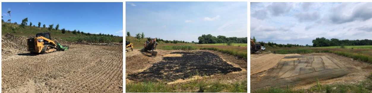
Figure 26. Infiltration basin retrofit and amended with biochar DelDOT US301, Delaware.
