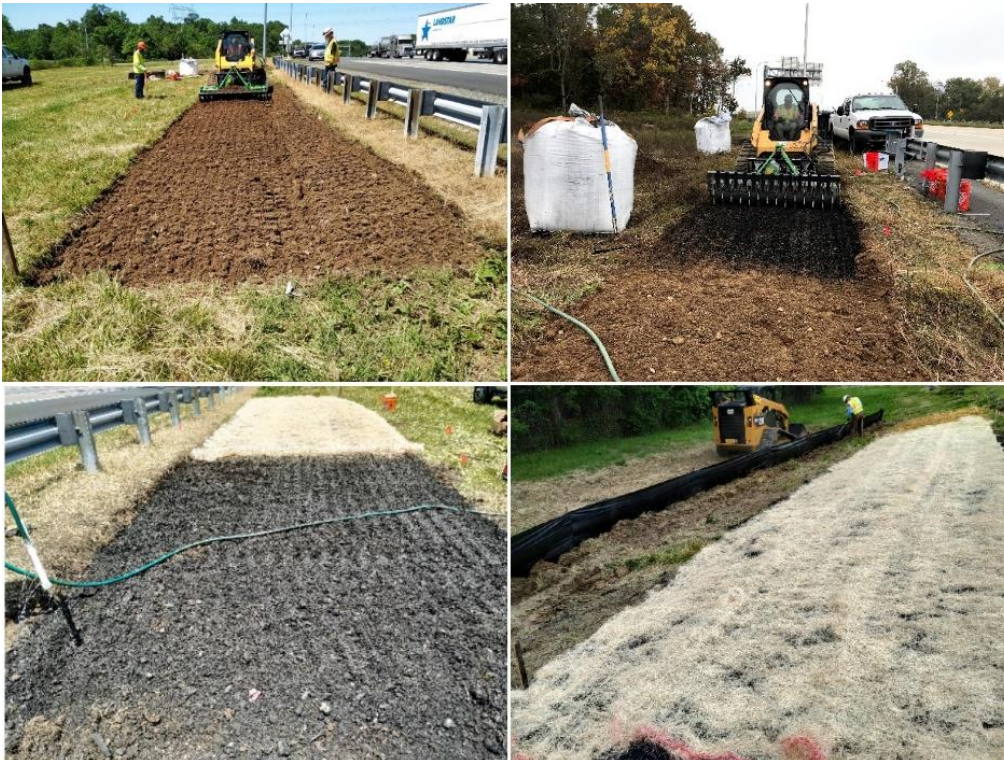
Figure 24. Biochar Amended Highway Greenway – 4% by mass. Similar benefits are at 2-3% by mass based on in-situ soil characteristics, as in Delaware and Maryland.
