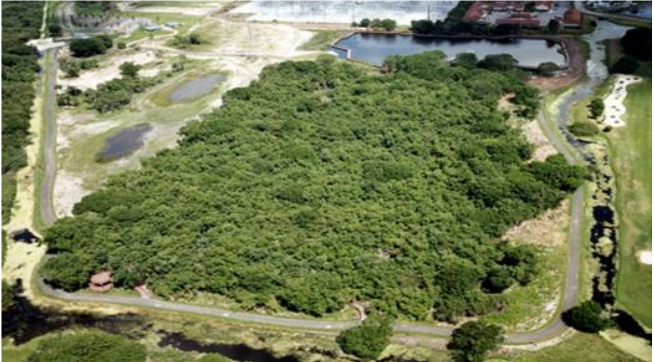
Figure 2. Large Regional Stormwater Treatment System
