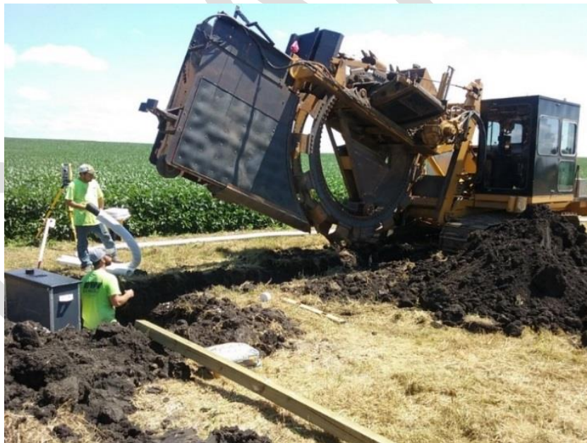
Figure 14. Installation of a saturated buffer. Source: USDA ARS 2015. Photographer: Dan Jaynes.
