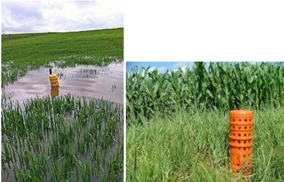
Figure 3. Surface tile risers for draining surface water from poorly-drained depressions (Left image from USDA-ARS magazine; right image from Scarve.net)
