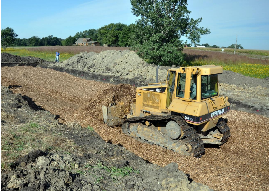
Figure 4. Source: USDA NRCS 2011, Flickr. Photographer: Jason Johnson. Installation of denitrifying bioreactor
