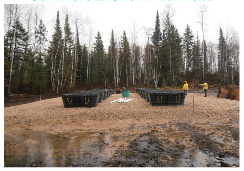
NSF 245 gravity treatment box + gravity trench
