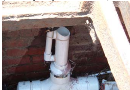
Figure 6. Example of inlet sampler to collect first flush samples (courtesy City of Baltimore)
