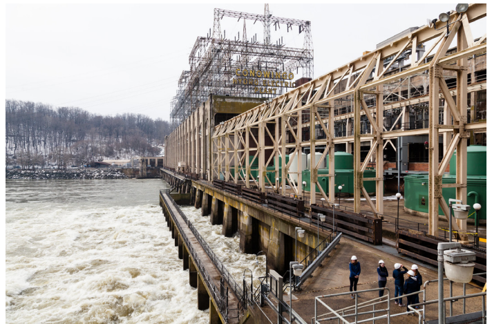
The Susquehanna River flows strongly past the Conowingo Dam near Conowingo, Md., on March 11, 2015. With earlier snow melt, roughly 85,000 cubic feet of water was flowing through the dam every second that day, and all 11 turbines were in operation, generating roughly 490 megawatts of electricity. (Photo by Will Parson/Chesapeake Bay Program)
