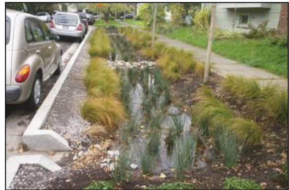
Figure 8 – Typical urban bioswale (Source: American Forests, 2012)
