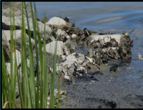
Figure 3. Oysters colonizing appropriately-sized granite on the sill below Mean High Water.
