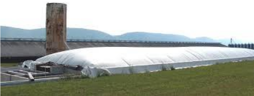
Figure AD.2. Plug Flow Anaerobic Digester Located on the Schrack Family Dairy Farm in Clinton County, PA (Penn State Extension).
