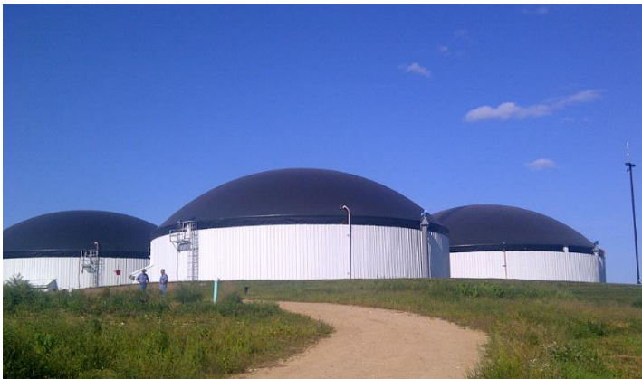
Figure AD.1. Complete Mix Anaerobic Digesters Treating Dairy Manure Slurry and Food Waste near Madison, WI. (Oklahoma Cooperative Extension Service).
