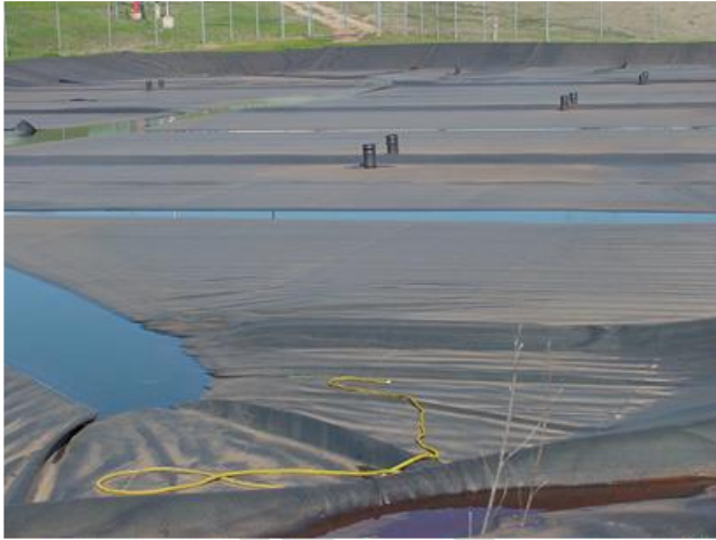
Figure AD4. First Cell of a Covered Lagoon Digester System Located on the Oklahoma State University Swine Research and Education Center (Oklahoma Cooperative Extension Service).
