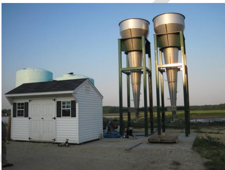
Figure WCT5. Demonstration of the Latest Generation of Cone Struvite Crystallizer on a Dairy Farm near Massey, Maryland (Sassafrassriver.org).
