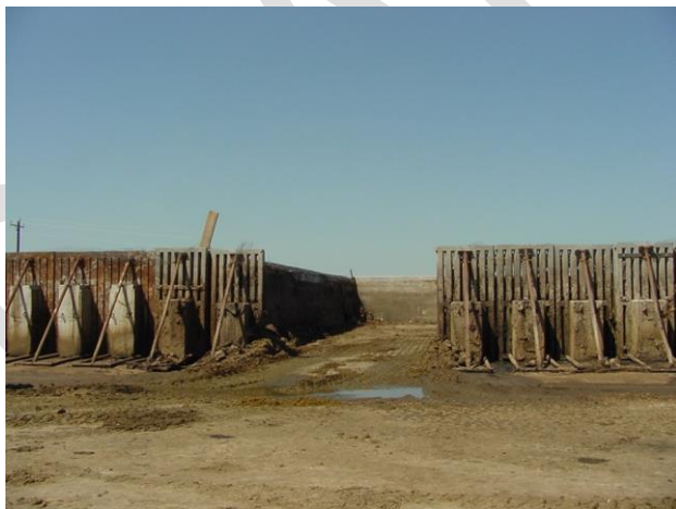
Figure STTL.5. Weeping Wall Storage Basin on a Large Dairy Farm in Erath County, Texas The Porous Dam has been Opened for Sludge Removal (YouTube:OSUWasteManagement).
