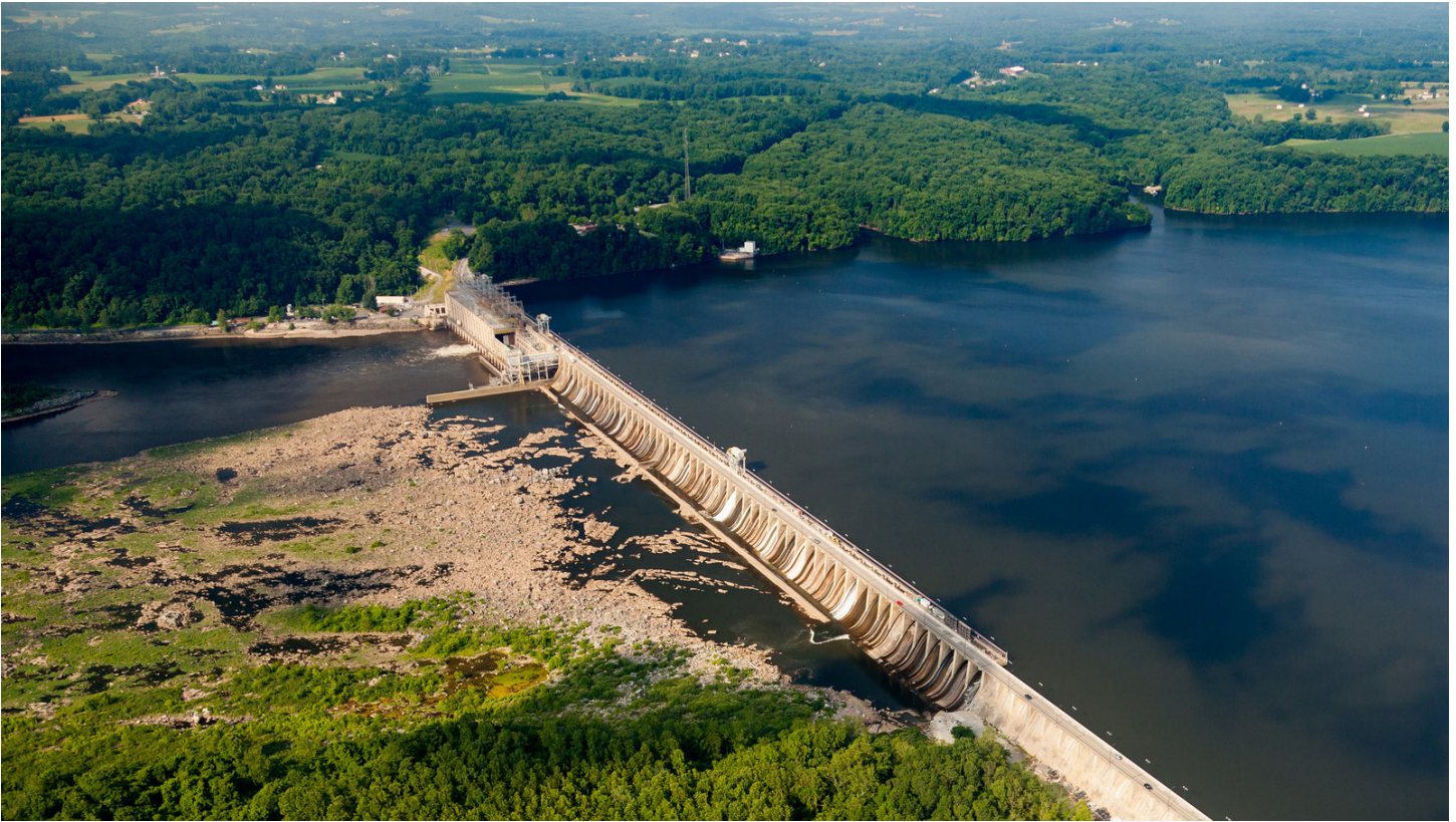
The Susquehanna River flows south past Conowingo Dam, toward Havre de Grace, Md., on June 27, 2016. Conowingo Dam has long trapped sediment runoff originating from farms and other sources upstream. But its capacity is reaching equilibrium, meaning it is trapping less sediment and sending more of it to the Bay.
