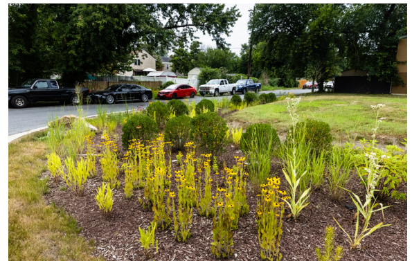
A rain garden sits at the intersection of Ingraham Street and Lafayette Place in Edmonston.
