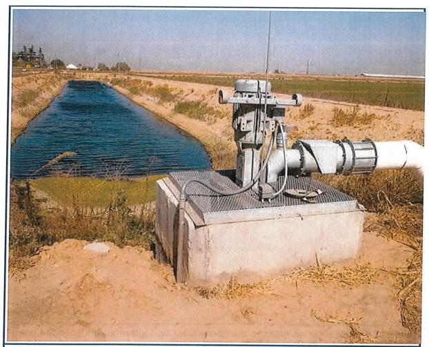
An irrigation tailwater recovery system in California. Note the recovery pond, the pond-outlet sump and the redistribution pump and piping. Image courtesy of USDA, NRCS.
