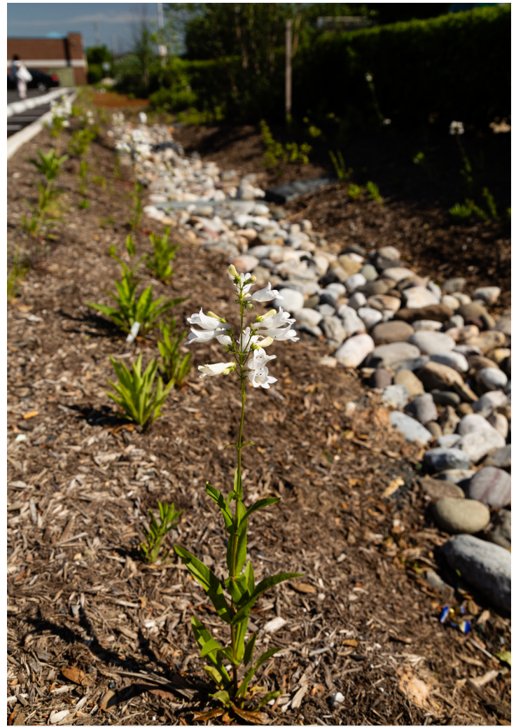
Plants placed between impervious surface area and the drainage channel will help to absorb and slow the flow of stormwater. Photo by Will Parson/Chesapeake Bay Program.
