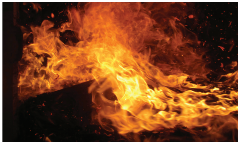
Wood chips and poultry litter burn in the combustion chamber of the bio-burner. (Photo: Glenn Rodes)
