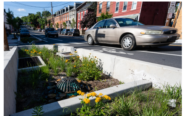
A vegetated curb extension filters stormwater while calming traffic and protecting a crosswalk.
