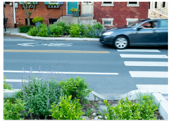
Curb extension captures and filters stormwater while calming (slowing) traffic.
